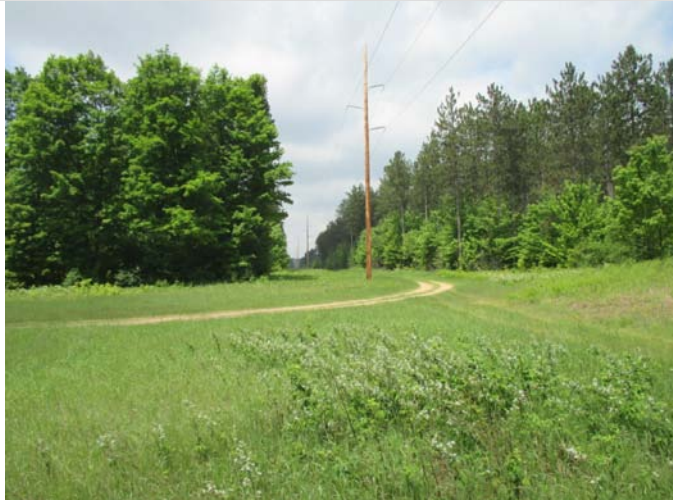
1. A view of the power line right-of-way on the north side of the site looking northwest.
