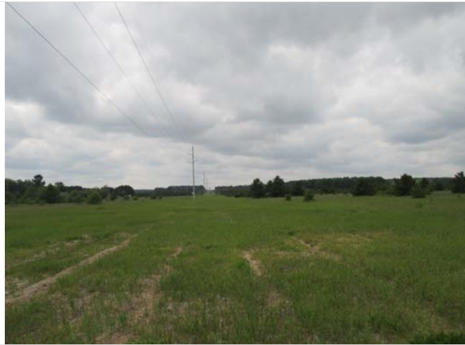
3. A view of the power line right-of-way on the south side of the site.
